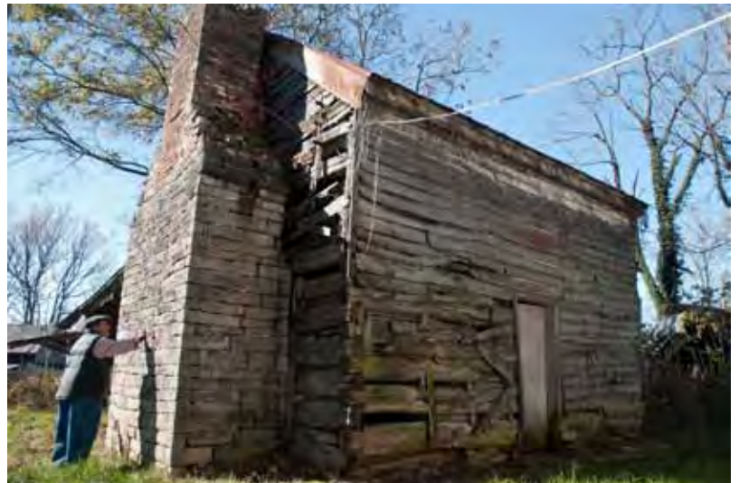
Duncan examines the workmanship of the cut stone used to build the chimney of Porter's original cabin, dated roughly between 1820 and 1830. In addition to the cabin, several other outbuildings still stand on the Porter farm.
